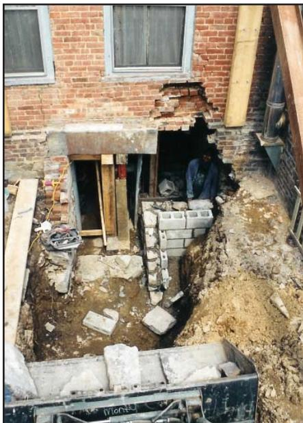
*Jack under lintel. Wall is rebuilt on concrete footing.*
