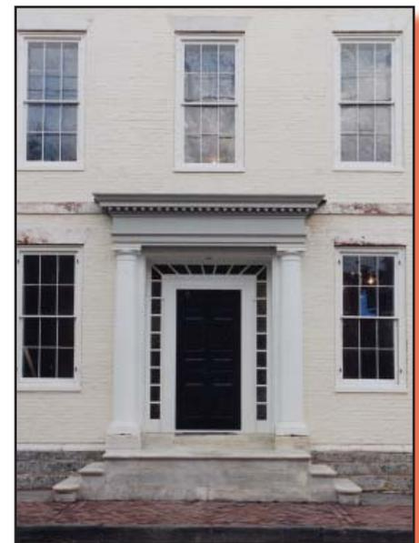
1803 townhouse with marble repaired and relayed on proper foundation. Entry restored to single doorway. Concrete sidewalk replaced with 19<sup>th</sup> century brick pavers.
