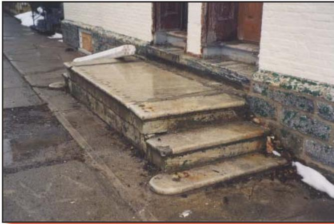
1803 townhouse. Marble entry in disrepair. Note concrete sidewalk has risen 8" from original grade burying bottom step
