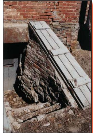
*Water blows out bulkhead wall. Lintel drops. Wall sags.*
